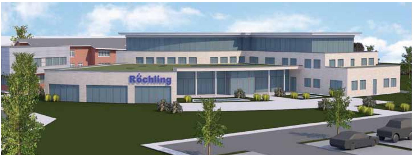
Under construction: The Industrial Center in Haren is set to be completed in autumn 2020; it will be home to large and representative conference rooms and new office rooms, and Corporate R&D will also have its home there
