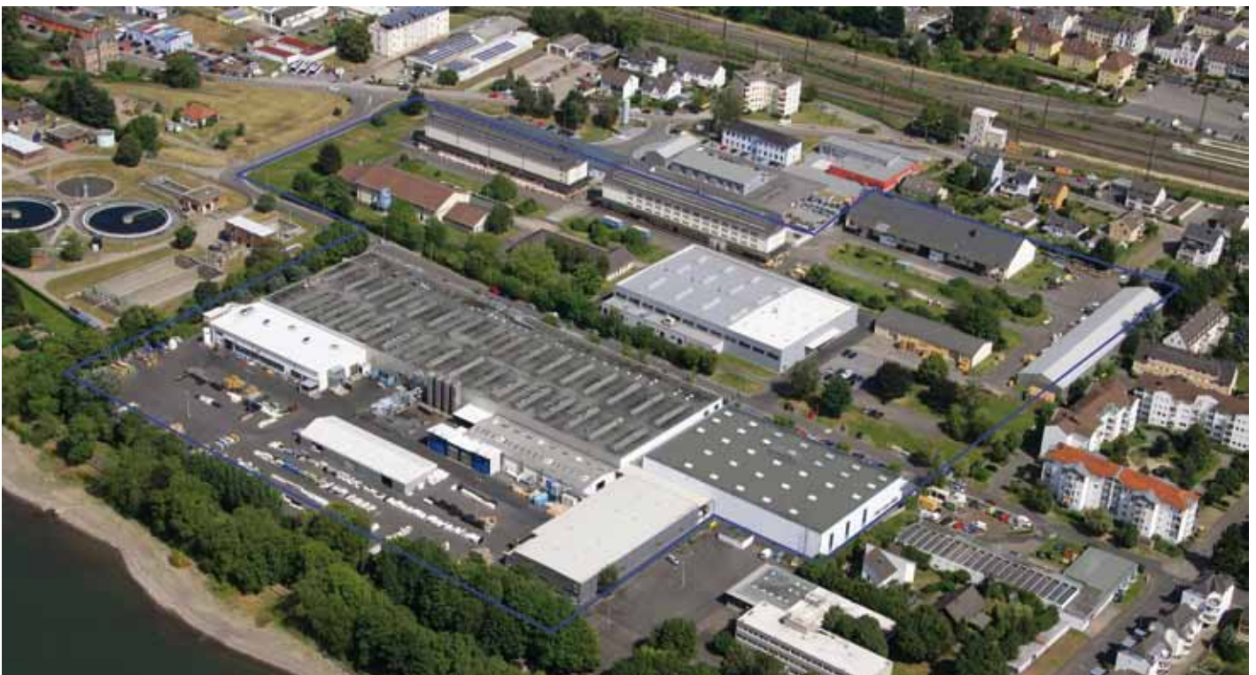
Centre of excellence for high-performance plastics: the Lahnstein site
